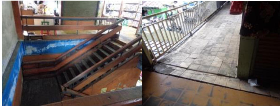
Figure 8. 2nd floor condition (Source: author)
