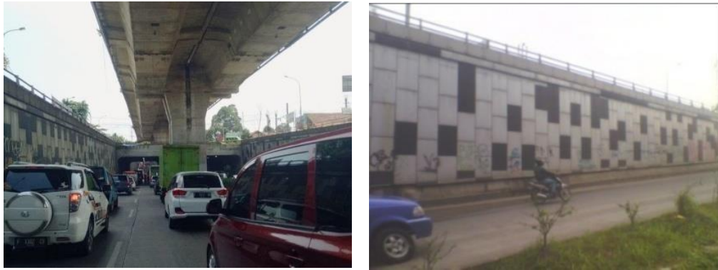
Picture 3. Traffic Jam and Vandalism in the Underpass
