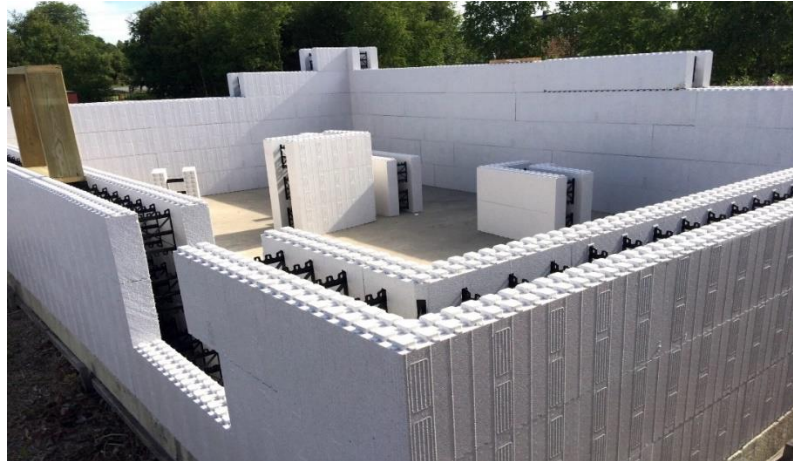
Gambar 2. sistem bangunan Insulated Concrete Formwork (ICF)
